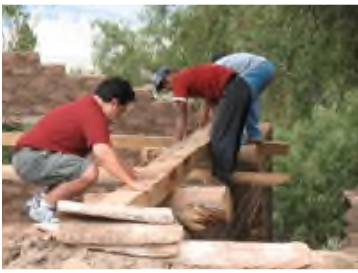
Building the church roof
